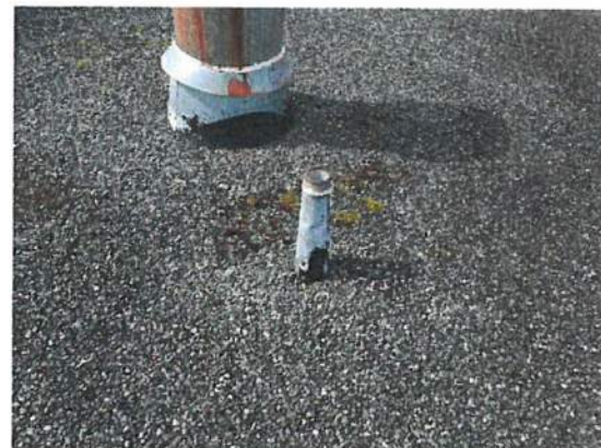
Photo 21: Tar – Roof on Vent (ND)
