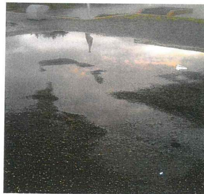
From the last photo, turning 90 degrees, facing flag pole, more pondling, added weight and improper drainage.
