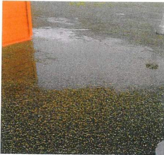
Roof adjoining old hose tower, more pondling, weight, pondling at seem of structure.
