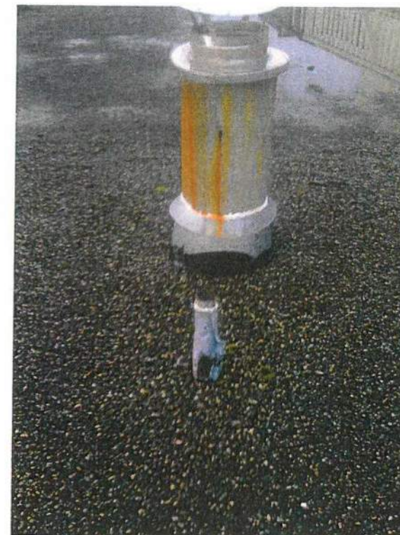
Some roof vents are need of repair or replacement.
