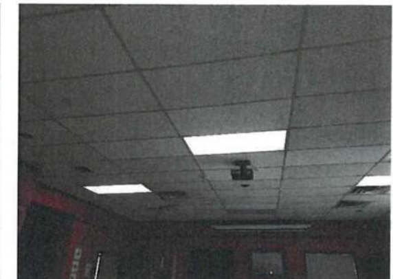
Fluorescent Light Ballast; Fluorescent Tube Lights (PCB; Mercury)
