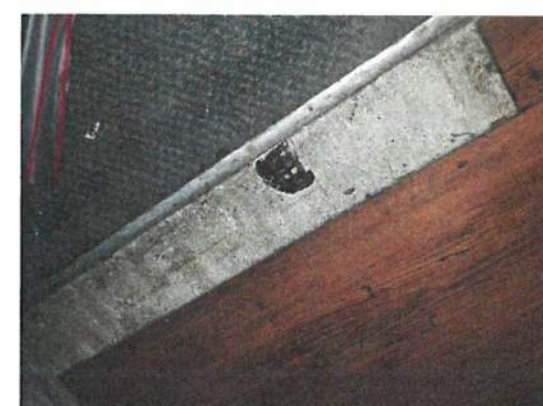
Photo 11: Vinyl Floor Tile – Banquet Hall Below Laminate (ND)
