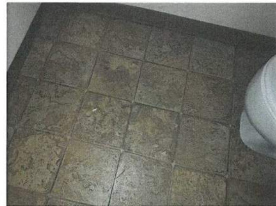
Photo 13: Sheet Vinyl Flooring – Washroom (ND)
