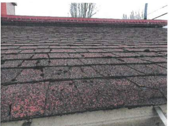
Photo 24: Composite Shingle – Gym Addition (ND)
