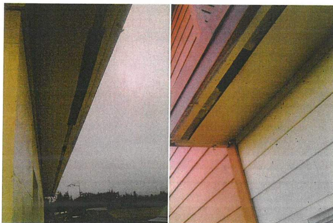
Roof venting, there are many fixes here with different types of methods, due to age, birds are making egress easily for nesting, etc..
