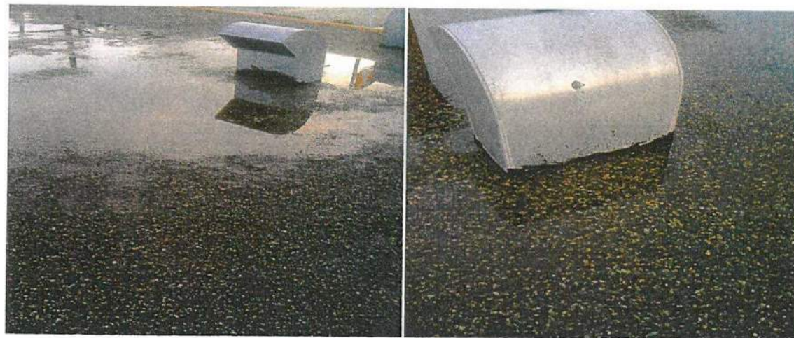
More pondling, the issue here the pondling is around HVAC outlets, which has possible egress to interior.
