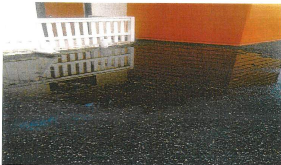
The pooling you see here is called "pondling", location here is outside the upper training room classroom. One of the issues here is the added weight of water on our structure, also improper location of drains.
