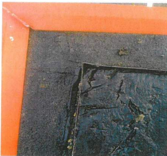
Exposed tar, no gravel to protect, cracks which make good egress of water to interior.
