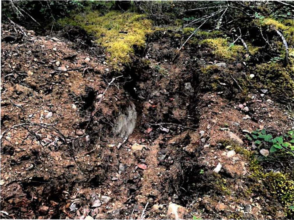
Photo 3. Example of test pit excavation.
